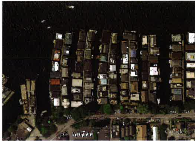
Figure 2-14. Non-Conforming Floating Homes.
